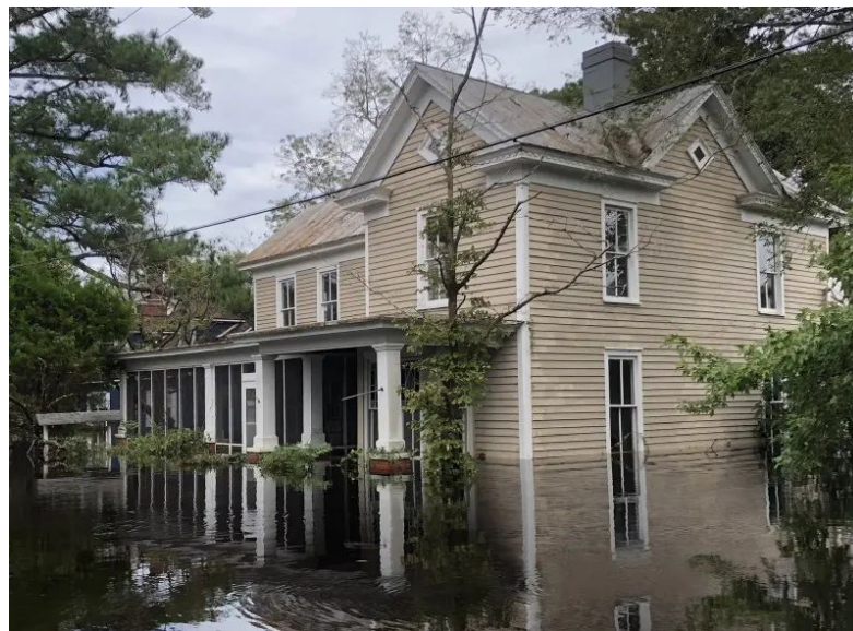
After flooding (photograph)
