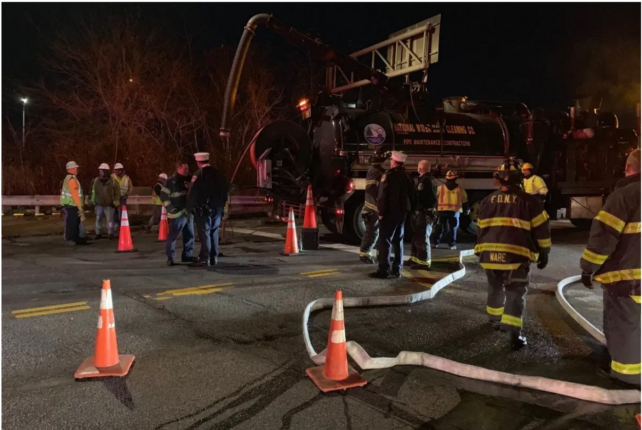
A clogged sewer line sent raw sewage flooding into the basements of dozens of homes in Southeast Queens in December 2019.
