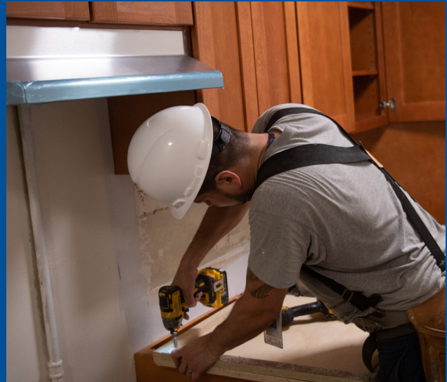
Repairs at NYCHA’s Betances Houses in the Bronx.
