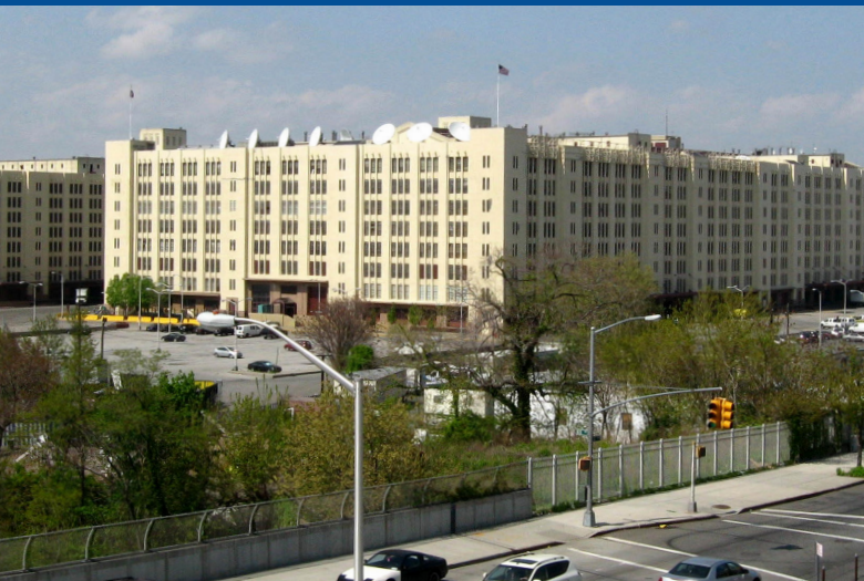
Brooklyn Army Terminal, location of the Sunset Park Solar community-led solar project.
