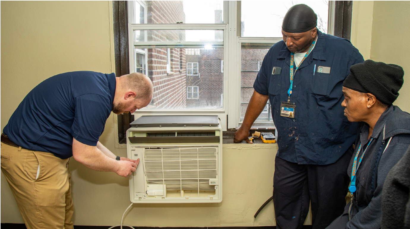
Installing a heat pump window unit at Woodside Houses as part of NYCHA's Clean Heat for All program. Source: NYCHA
