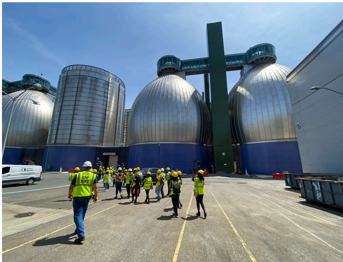
Since 2016, the City operates a full-scale co-digestion program at the Newtown Creek Wastewater Resource Recovery Facility to turn wastewater biosolids into renewable energy. Source: Mayor's Office of Climate & Environmental Justice
