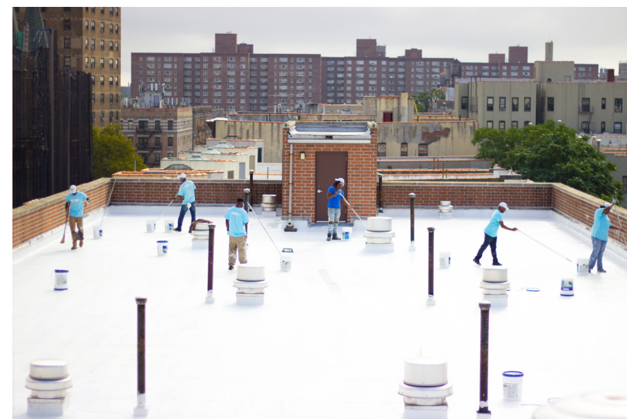
Spray showers are found at many of the City’s public playgrounds (top and middle). NYC CoolRoofs provides New Yorkers with paid training and work experience installing energy-saving reflective rooftops (bottom). Source: Department of Environmental Protection; Mayor’s Office of Climate & Environmental Justice
