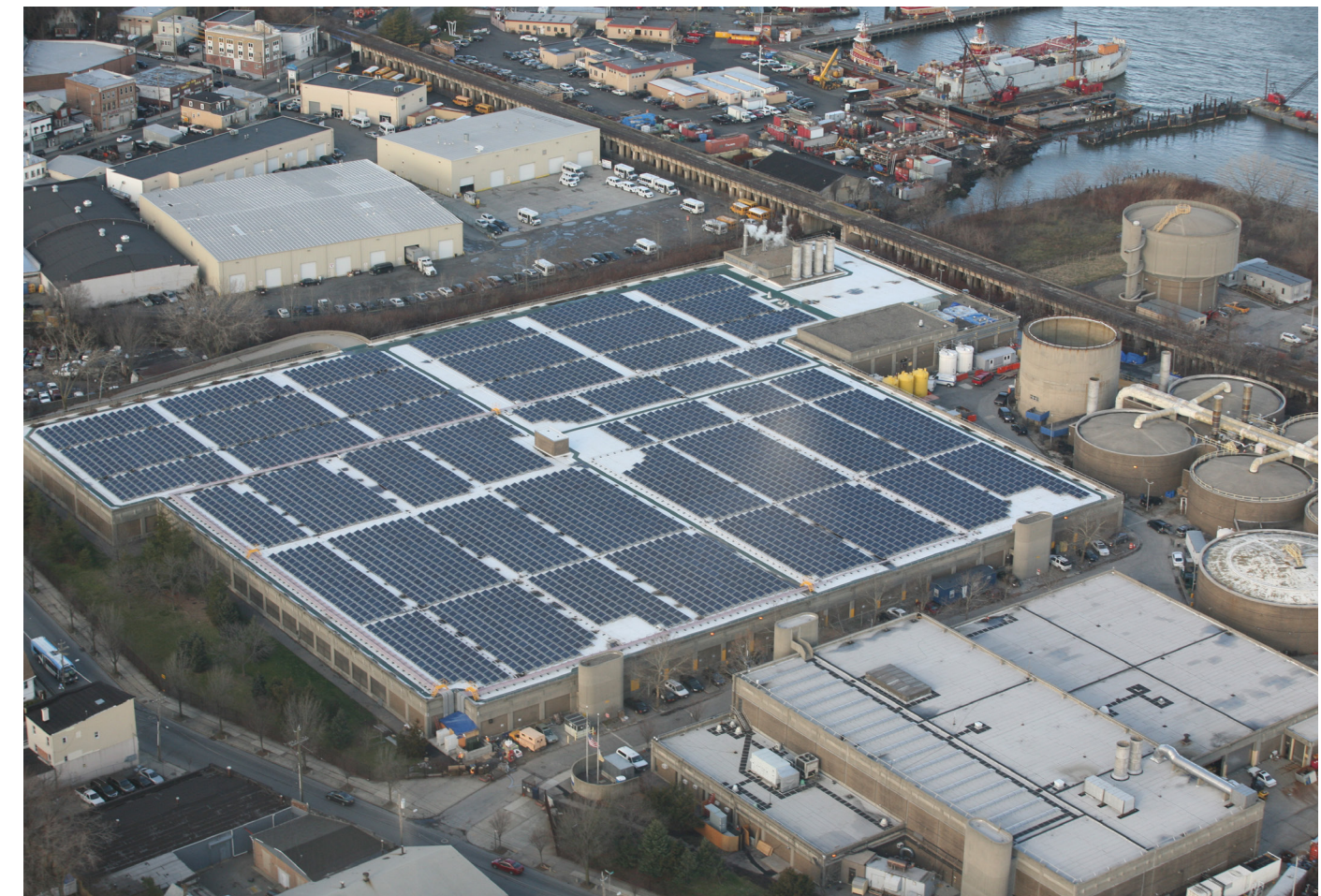
Solar panels installed on the roof of the City's Wastewater Resource Recovery Facility in the Port Richmond neighborhood of Staten Island. Source: Department of Environmental Protection
