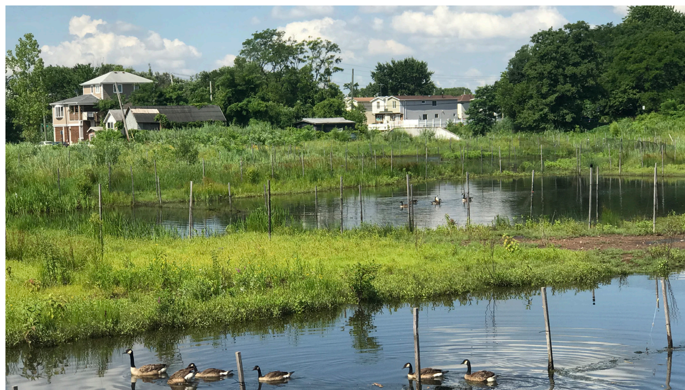
The New Creek Bluebelt was constructed to protect residents of Midland Beach, Staten Island from flooding. Source: Mayor’s Office of Climate & Environmental Justice
