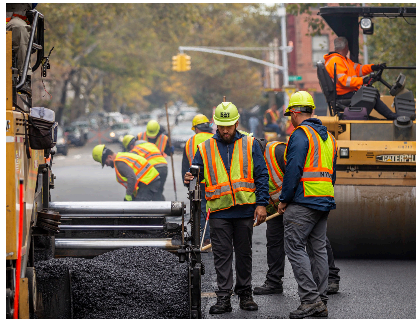
Road paving in Crown Heights, Brooklyn. Source: Department of Transportation
