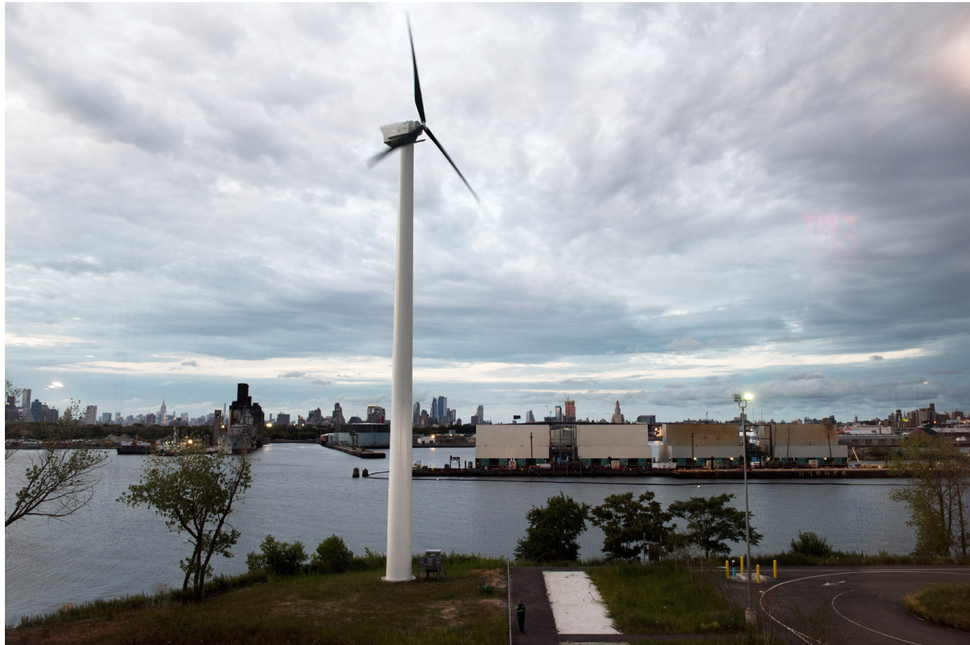
A wind turbine at the South Brooklyn Marine Terminal will help power a recycling plant. Source: NYC Economic Development Corporation
