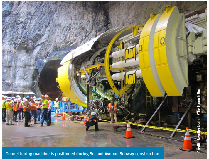
Tunnel boring machine is positioned during Second Avenue Subway construction
