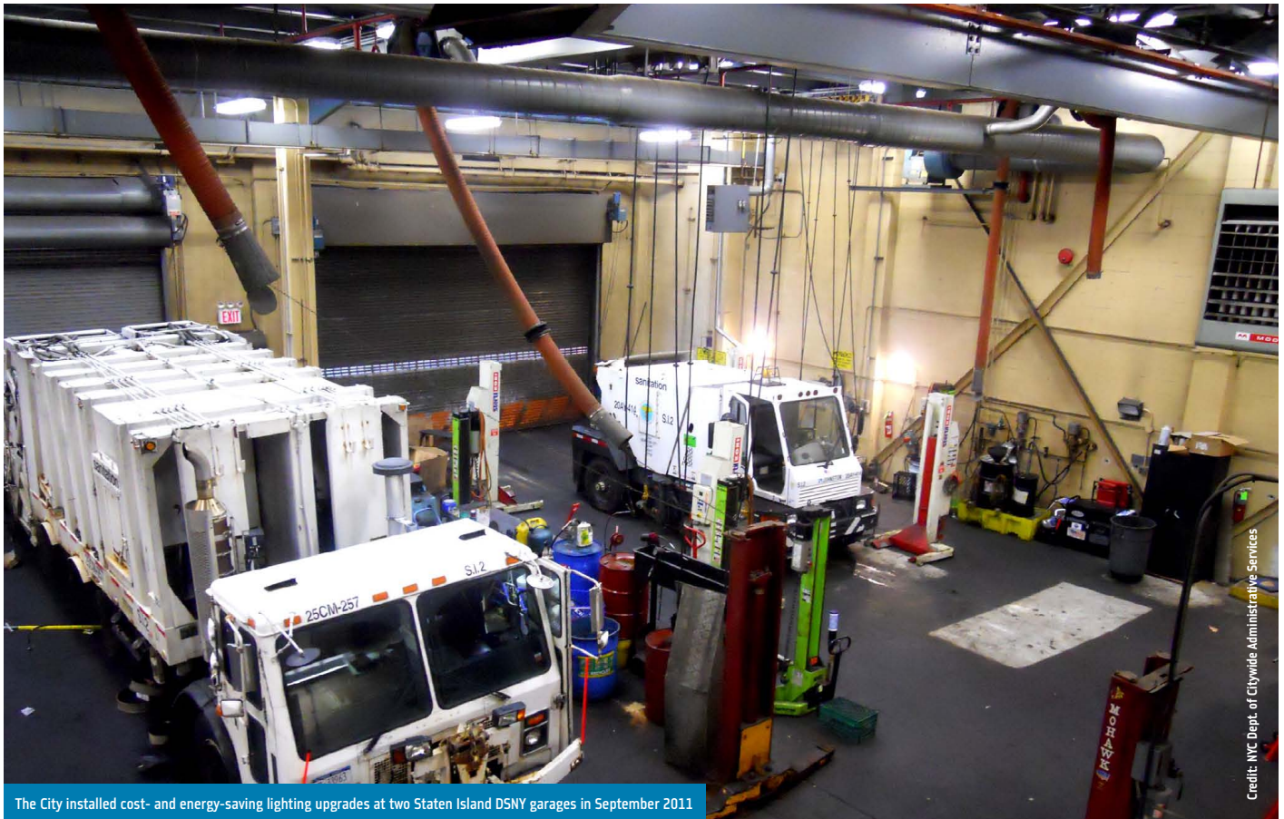
The City installed cost- and energy-saving lighting upgrades at two Staten Island D5NY garages in September 2011
