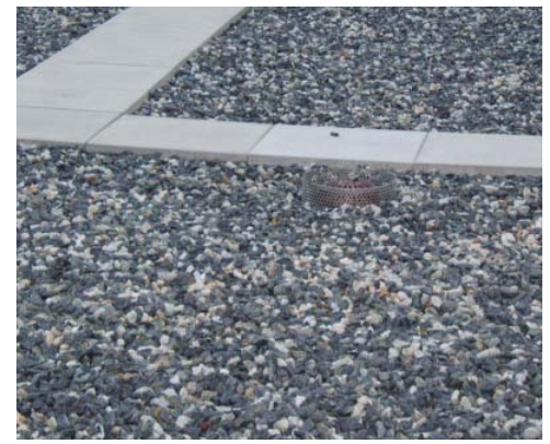
SCA Blue Roof on PS 12 Credit: NYC Department of Environmental Protection
