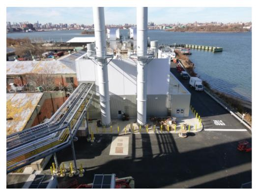
CHP uses waste heat from the electricitygenerating process to produce steam for heating, which makes such systems more efficient than boilers. The new CHP facility underway at Rikers Island will include two 7.5 megawatt (MW) combustion turbines with heat recovery steam generators, for a total of 15 MW installed capacity. The facility will generate nearly all of the electricity and steam needed to serve Rikers Island, and is projected to save the City nearly \$7 million annually.
