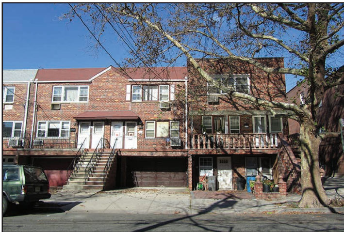
Figure 4.3 Attached Home in Canarsie with a Residential Unit on the Ground Floor
