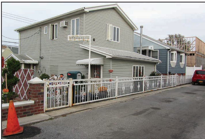
Figure 4.5 First Floor Below Street Level in Gerritsen Beach
